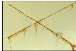
Common cold rolled sheet steel after a 336 hour salt spray test.
